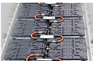
Battery charge/discharge test
